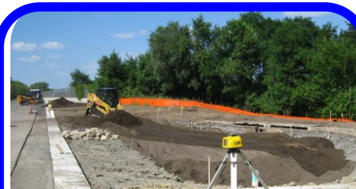
6" subdrains were installed. Backfilled with 70% coarse washed sand/30% compost
