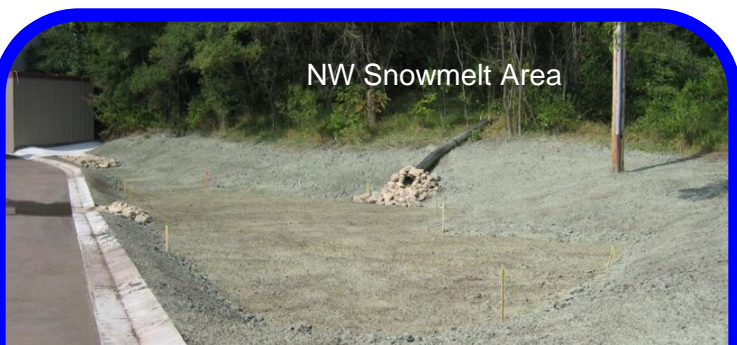
The NW snowmelt area is a 12" deep basin with compost amended in situ soils, 6" subdrains, and hydro seeded grass turf provides infiltration for volume reduction and treatment for arena ice shavings and snowmelt.
