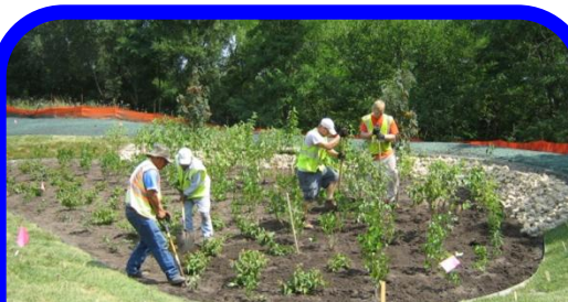
Native shrubs, metal edging, wood mulch and perimeter sod were installed
