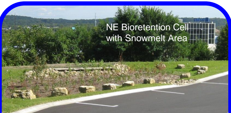
The NE and SE cells have a 3 foot depth of sand/compost media and 6" subdrains to provide biofiltration treatment. Temporary pool depths are limited to 12 inches maximum.
