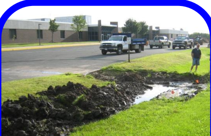
Hand excavated borings indicated there was more permeable granular soil two to three feet below the topsoil.
