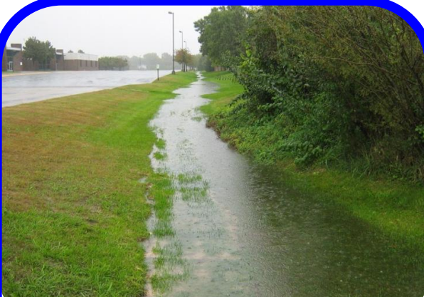
Amended soil turf Infiltration area during a rain event. Surface ponding completely infiltrated within six hours following the rain event.
