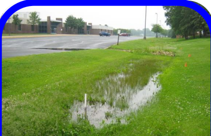
An existing 1,320 foot long drainage swale with poorly draining soils provided little water quality treatment .
