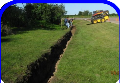
Soils were replaced in a 330 feet long trench to create 1,320 square feet of infiltration on the one side of the swale.
