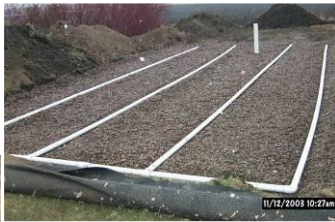
Replacing a septic tank and drain field
