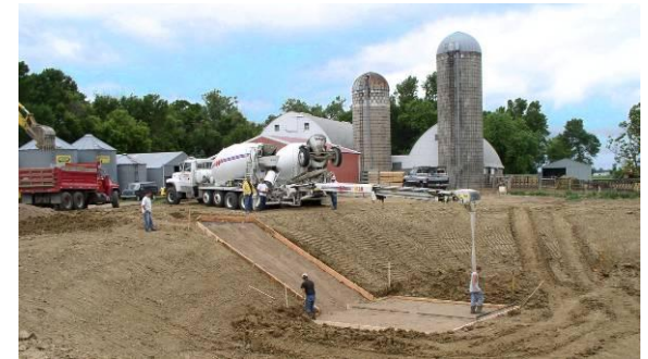
Feedlot improvements under construction
