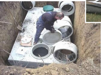
Replacing a septic tank and drain field
