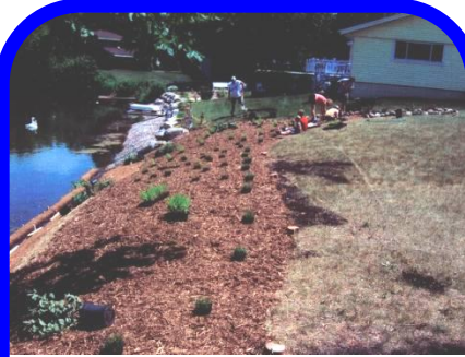
Installation of native aquatic, transitional, and upland plants and shrubs
