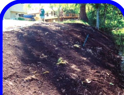
Repair of eroded areas and soil amendments
