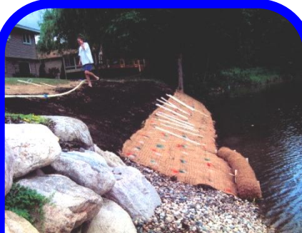
Installation of erosion control blanket and coconut fiber biologs
