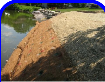
Bank after installation of erosion control materials
