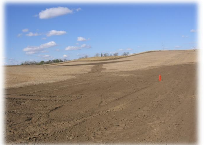
Completed Basin 3 and Basin 4.
