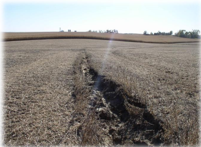
Gully erosion prior to construction basin 3 and Basin 4.
