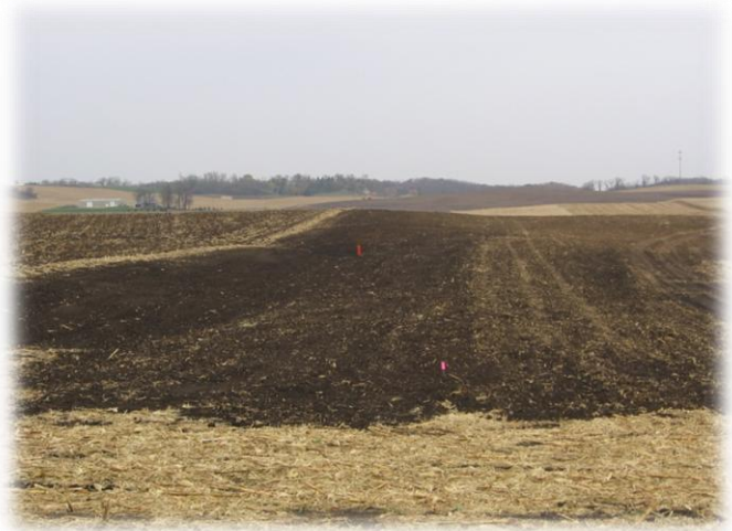
Completed north water and sediment control basin
