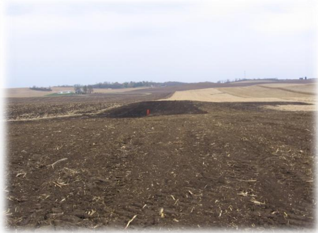
Completed south water and sediment control basin
